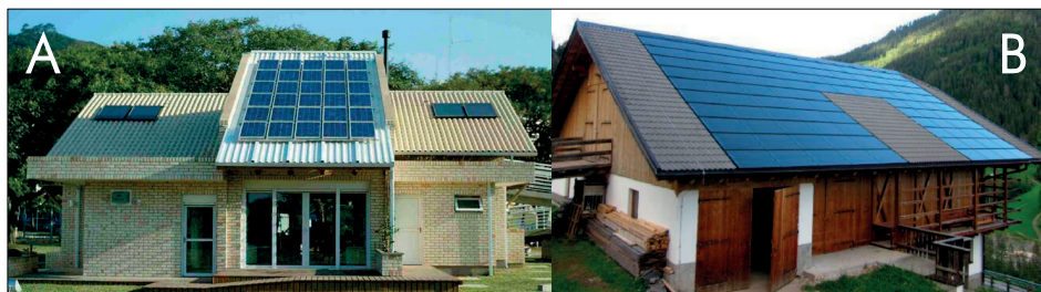
Figure 1. Photograph of rooftop BAPV realized in Florianopolis, Brazil (A) [5] and photograph of rooftop BIPV realized in Badia, Italy (B) [6].
